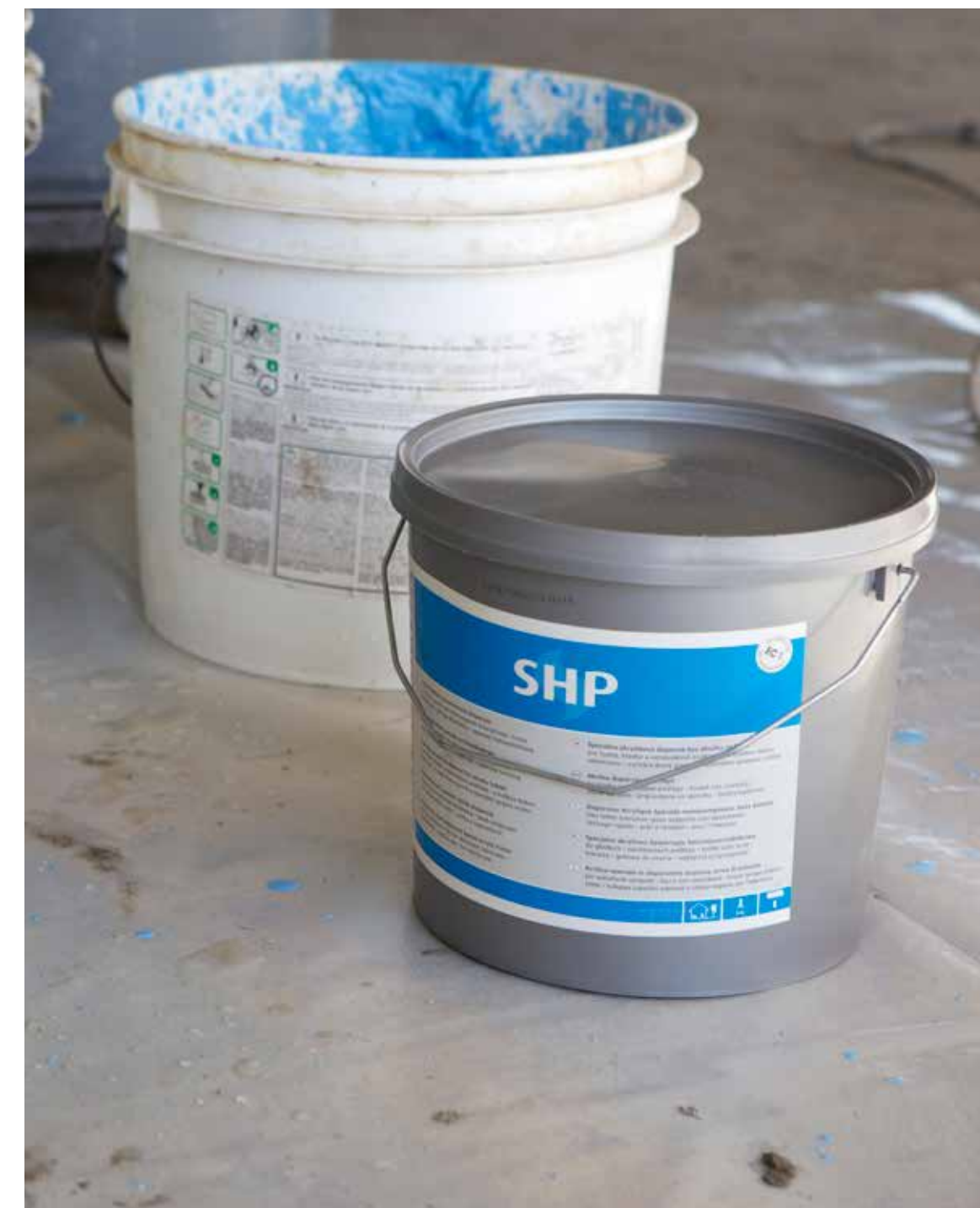
Priming reduces absorption by the substrate, protects sensitive subfloors, binds residual dust, and improves adhesion of the leveling compound.
