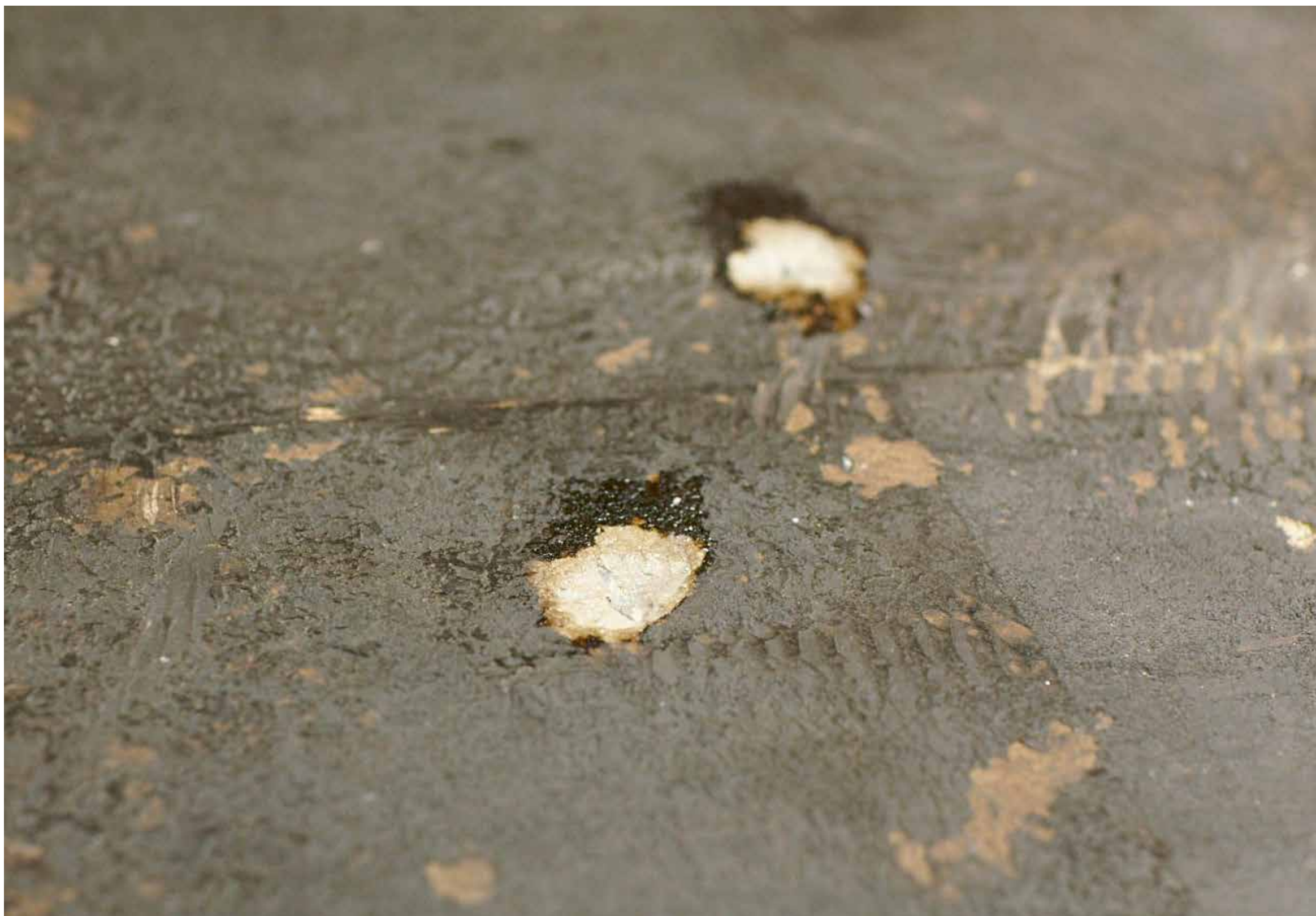
The prior floor covering was removed leaving the exposed concrete and residual cutback adhesive.
