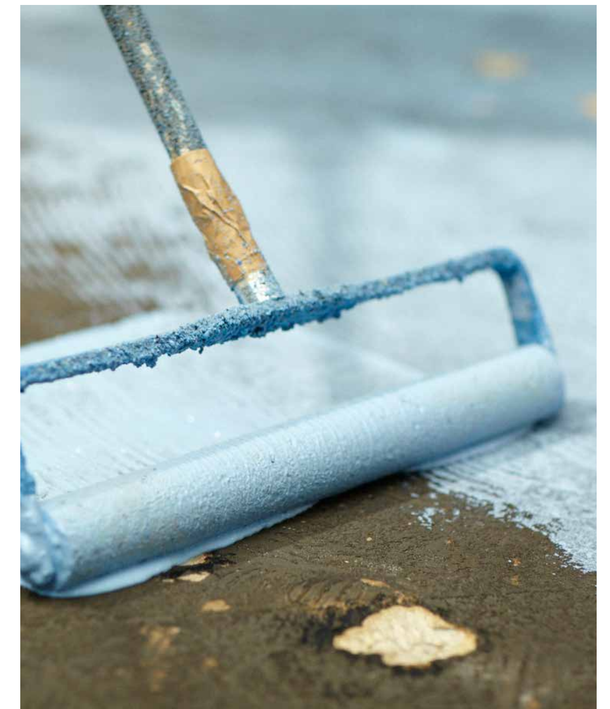
Schönnox SHP is ideal for use on interior non porous substrates drying in only 1 to 2 hours.
