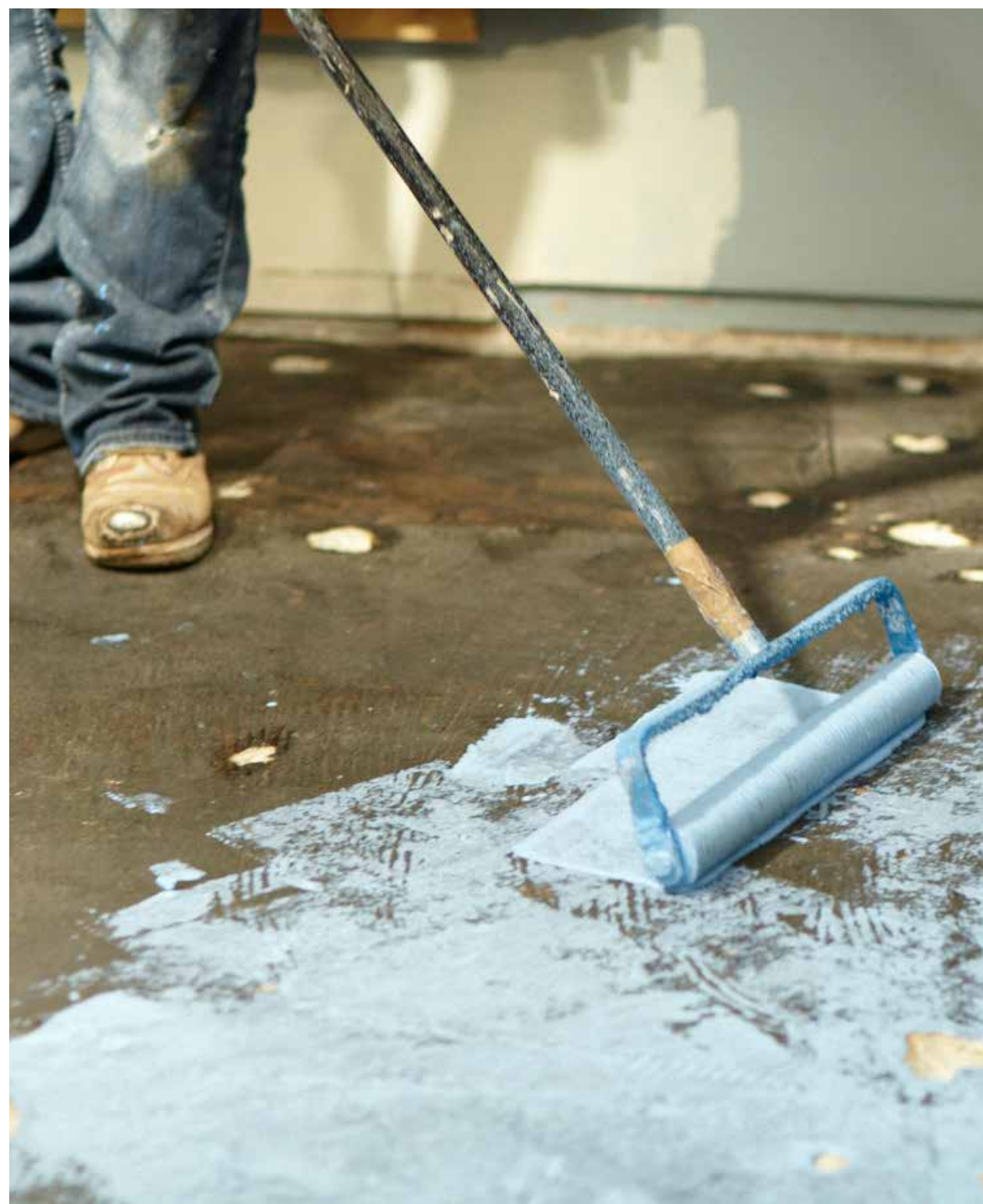
Schönnox SHP, special acrylic primer, is applied from a standing position with a low nap roller.
