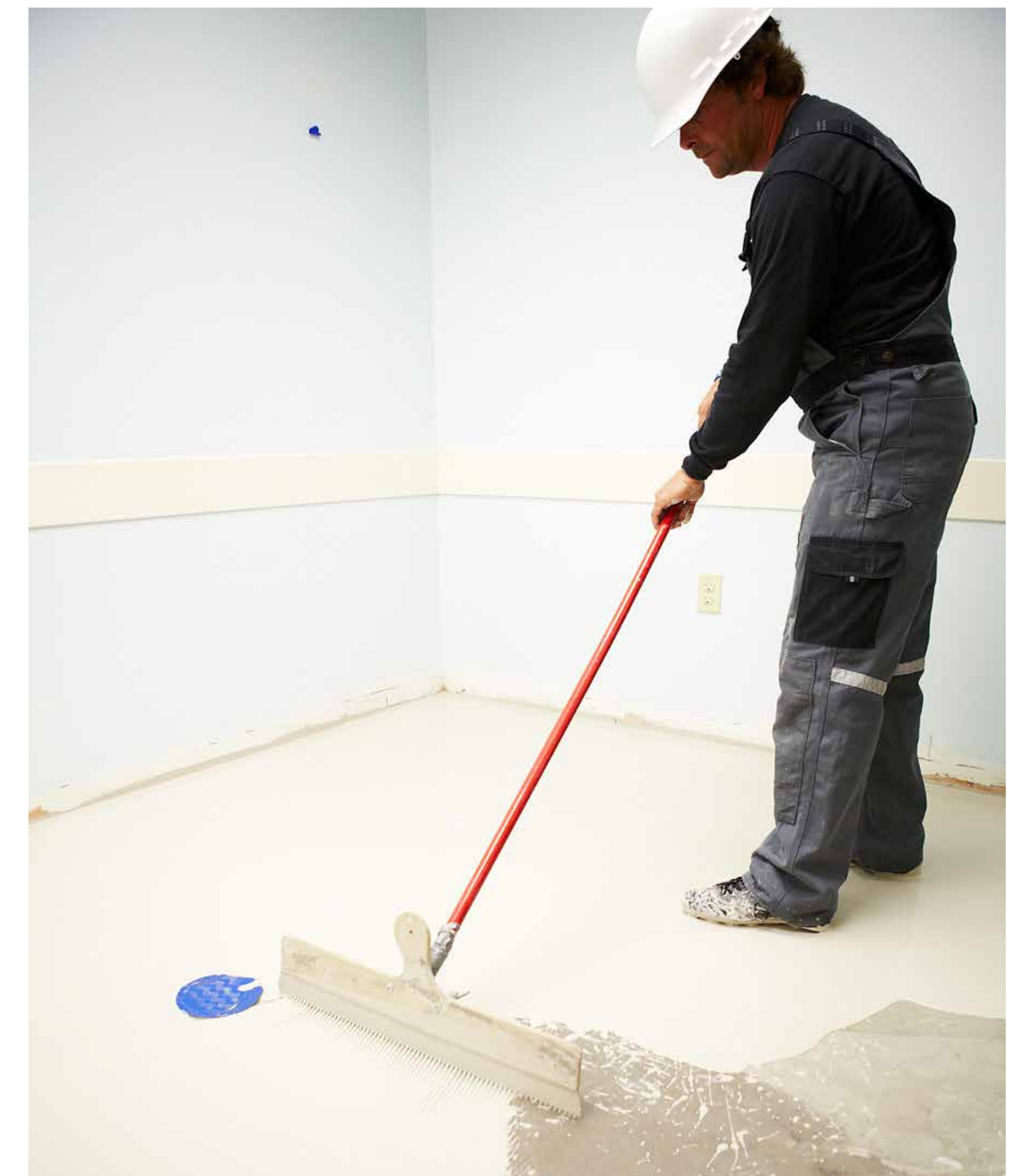
High polymer content gives Schönox AP excellent self-leveling capabilities and flow characteristics with minimal installation time ensuring smooth, flat subfloors.
