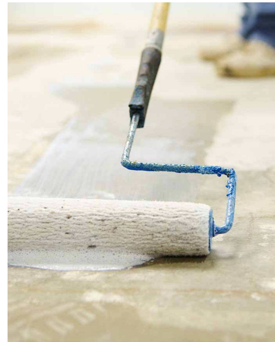
Schönnox VD is applied using a 3/8" nap roller.
