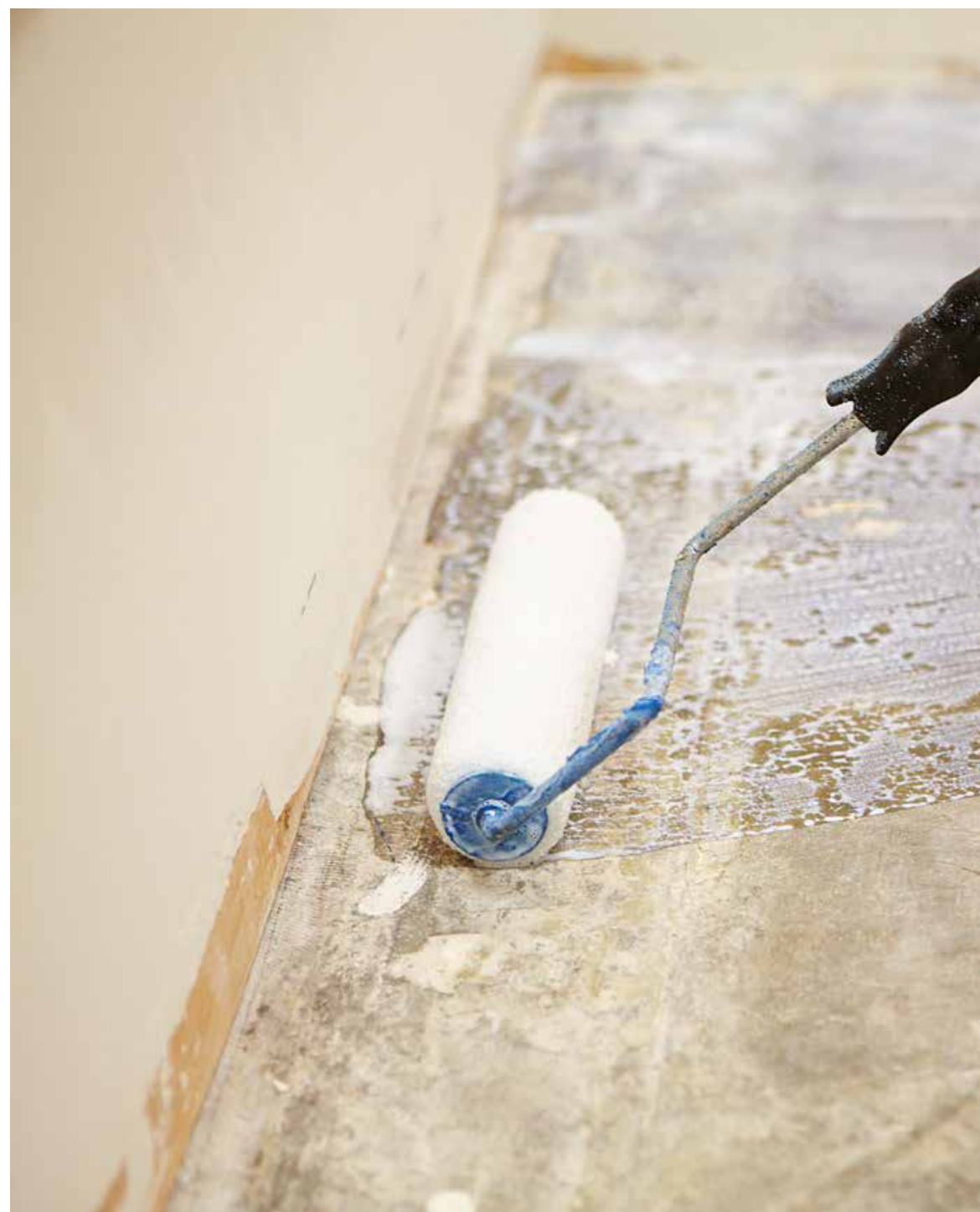
Schönnox VD is a universal acrylic primer for use prior to applying Schönnox underlayments.
